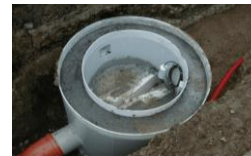
socket Parshall flume
